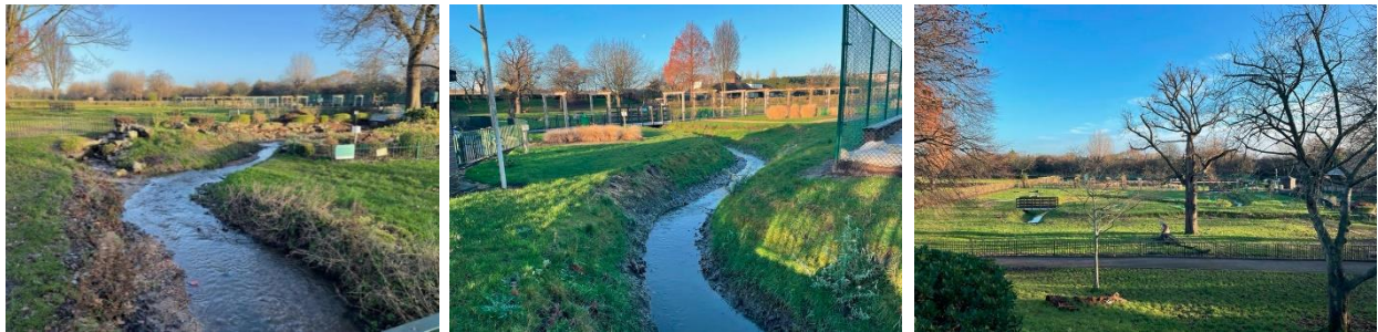
Wimbledon Park Brook River Restoration and Deculverting Project, Wimbledon Park 2022
